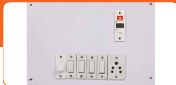
Screw mount its front plate on the switchboard.
